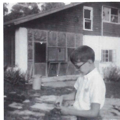
Original Dining Hall & Kitchen
